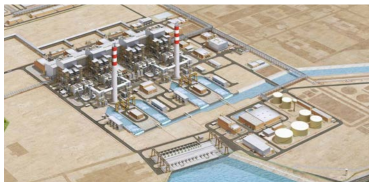
Jeddah South Thermal Power Plant Stage-1
