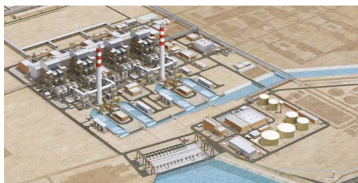
Jeddah South Thermal Power Plant Stage-1
